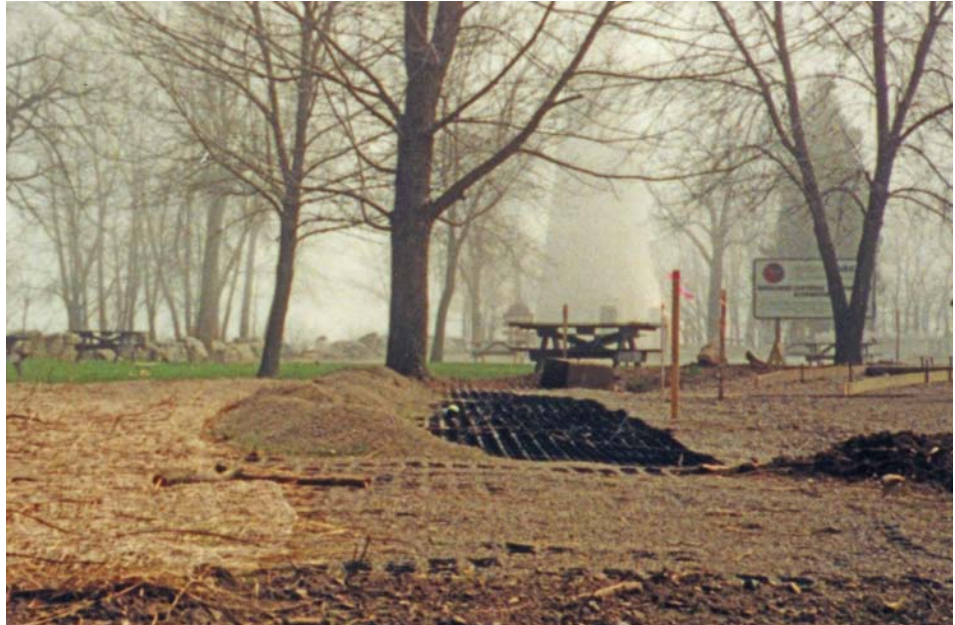
Pervious Paver installation
